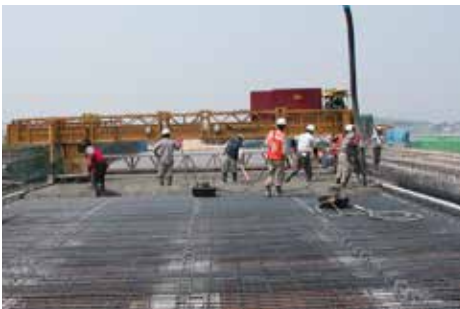
Installation of Sinnae Bridge Slab Concrete (Jeongeap~Taein)
