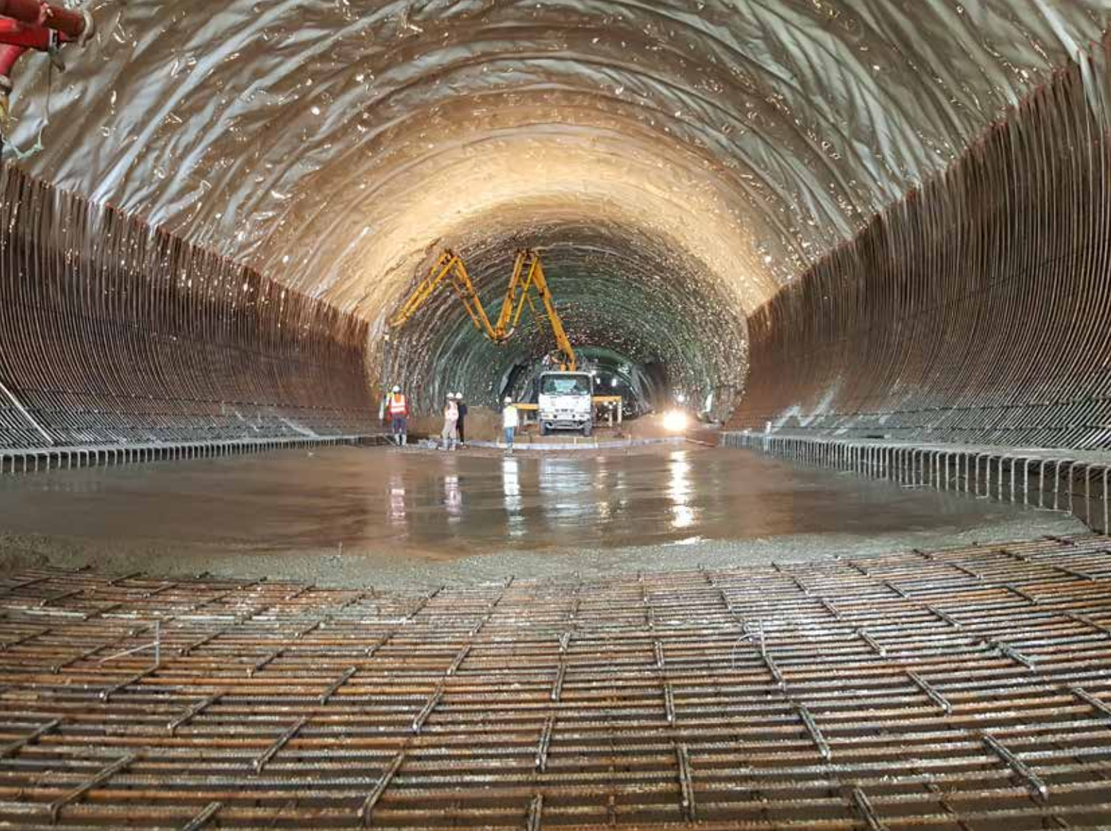
Installation of Tunnel Invert (Seokdong~Sosa)
