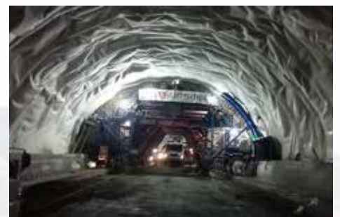
Installation of Tunnel Lining Concrete (Seokdong~Sosa)
