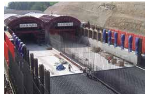
Inspection of Open-Cut Type Tunnel (Steel Industrial Complex Connected Road)
