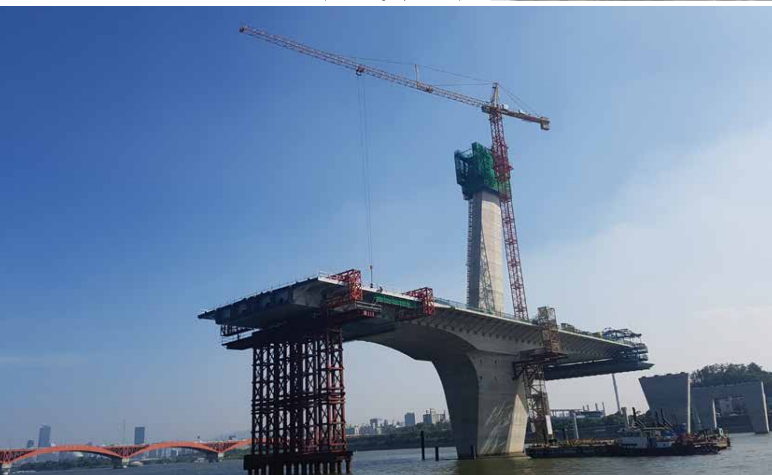
Construction of World-cup Grand Bridge (Pylon, Main Span)
